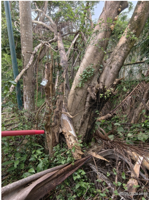
T202 - Decay Trunks (F)
